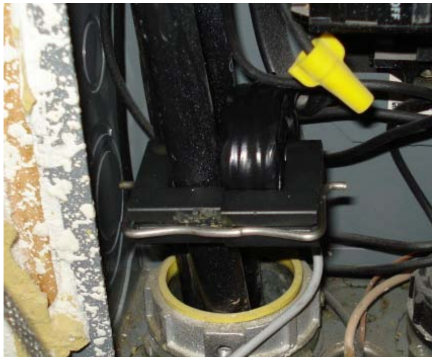
The current transformer sensors, one for each phase. They are installed in a way so that if they fall they won't short anything out.
